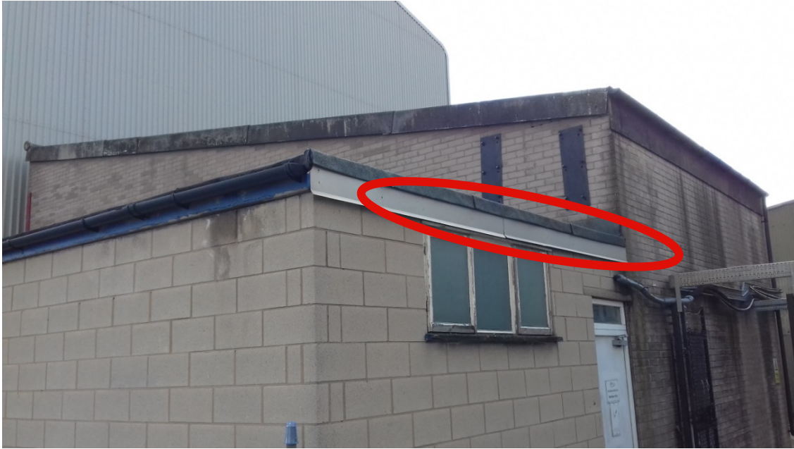
Photo 2 - Building 1, Development Parcel F
